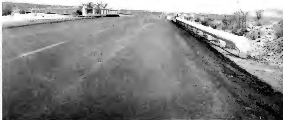
Another bridge approach protected by flared guard railing
